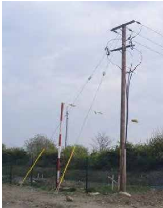
Figure 3-1: A typical MV line/cable interface pole
